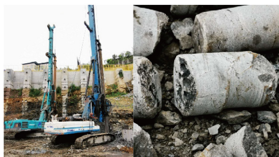
• Construction site in Chongqing
