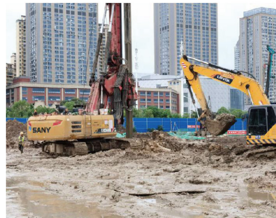
• Construction site in Wuhan Jiangxia
